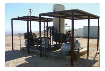
SCREW COMPRESSORS Figure 1. Such units are unrivalled for small applications. *Source: Accurate Air Engineering.*
