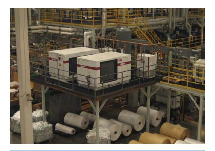
AIR COMPRESSOR MODULES Figure 3. Modular approach for turbocompressors can cut both capital and operating expenses. *Source: Accurate Air Engineering.*
