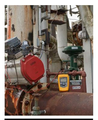
Figure 1. Smart electronics will control what essentially is a smart pressure regulator to increase or decrease pressure as needed to move the control element to the desired position.
