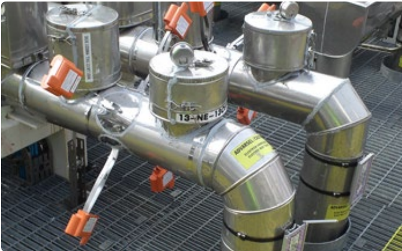
Figure 2. Installing multiple ultrasonic units (orange) in areas at elevated risk of internal corrosion can help spot localized attack.
