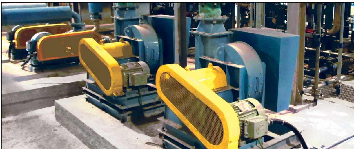
Figure 1. One blower is operating while the other serves as a standby.
