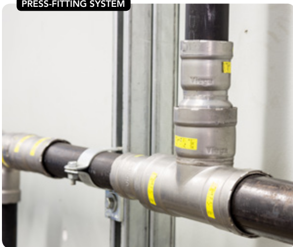
Figure 3. Using press-fitting technology saved an estimated 30% installation time over soldering.
