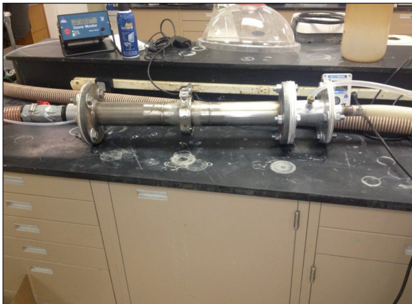
Piping used to pump ozone through lines
