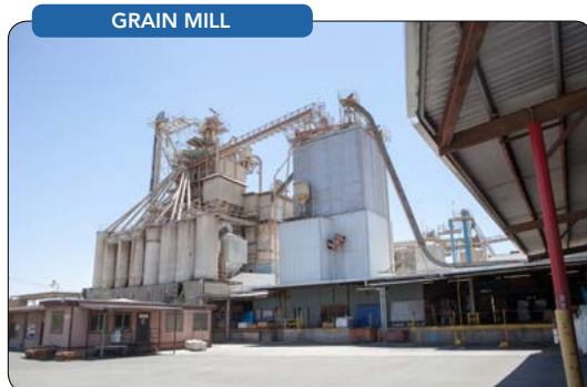
Figure 1. Star Milling’s facility includes a variety of equipment that produces tons of feed per day, generating large amounts of dust. Source: Air Cleaning Technology
