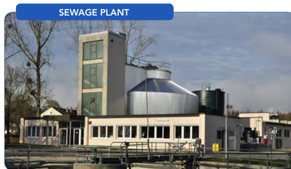
Figure 3. The Burghausen public utility company in Germany operates a sewage plant including sewage treatment and connected combined heat and power plant fueled by digester gas.
