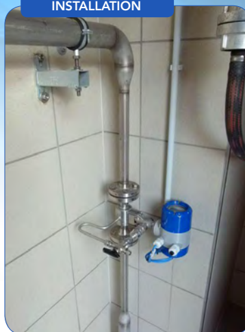
Figure 6. The Optiswirl vortex flowmeter from Krohne was installed with a flange connection in a descending pipeline.
