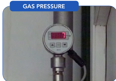
Figure 5. With the installation of a low-pressure system, the flowmeter still reads reduced gas pressures of just 7–8 mbar (0.10 psi).
