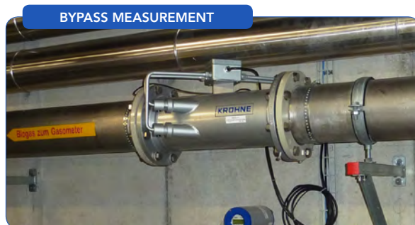
Figure 2. A Krohne GFM 700 ultrasonic device is used for a bypass measurement.
