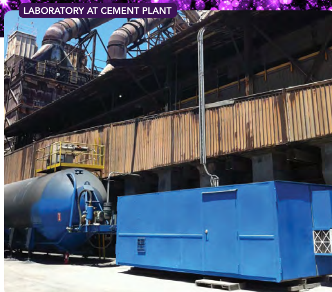
Figure 2. Vertical pipes provide laboratory (blue container) with flue gas directly from stack. Source: Oakbio.
