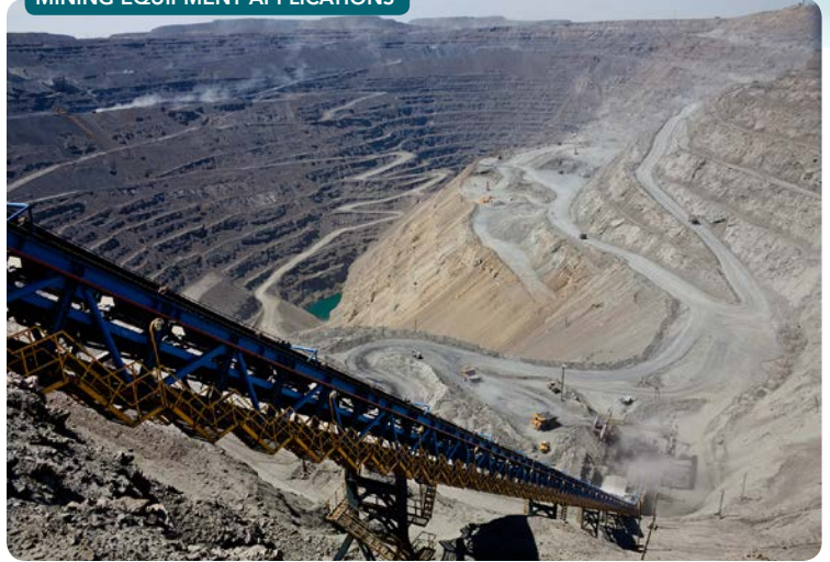
Figure 4. Medium voltage VFDs used in mining applications can improve speed control, lengthen maintenance intervals and lower the energy costs associated with operating the equipment.
