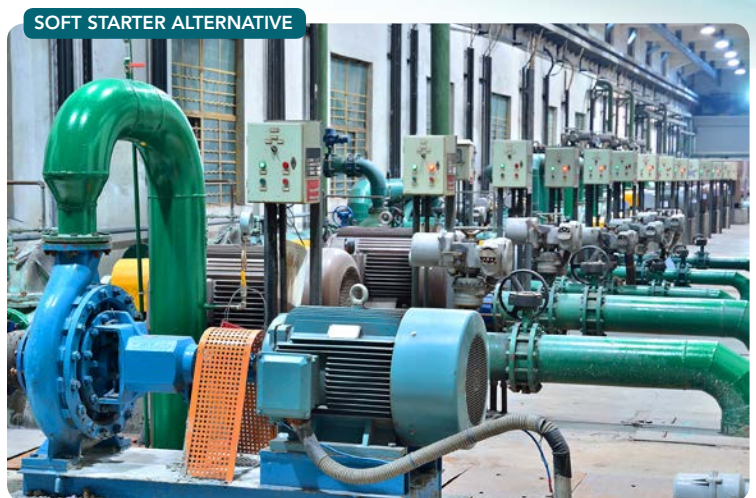
Figure 2. Variable frequency drives are inherently soft-starters. They ramp the voltage to the motor and limit inrush currents, prolonging motor life.
