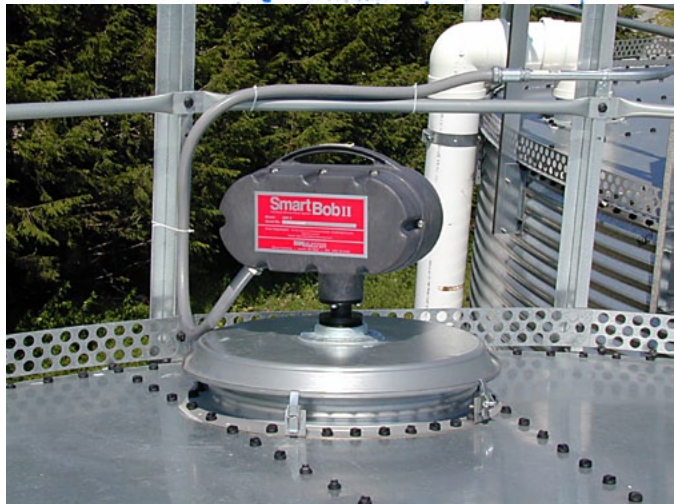
Figure 2. For the best accuracy, the sensor should be mounted on the roof of the silo about 1/6 of the way in from the outer perimeter.
