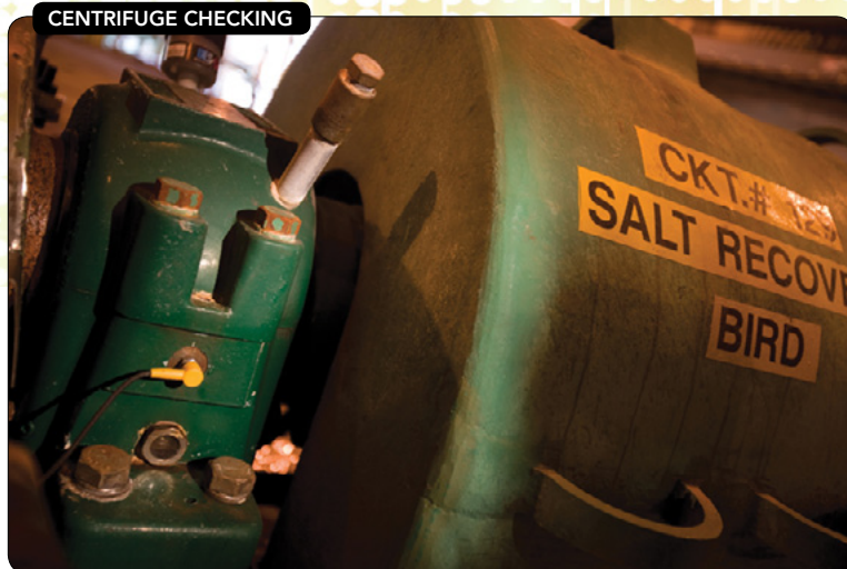
Figure 3. Wireless vibration transmitters monitor Salt Bird centrifuges.
