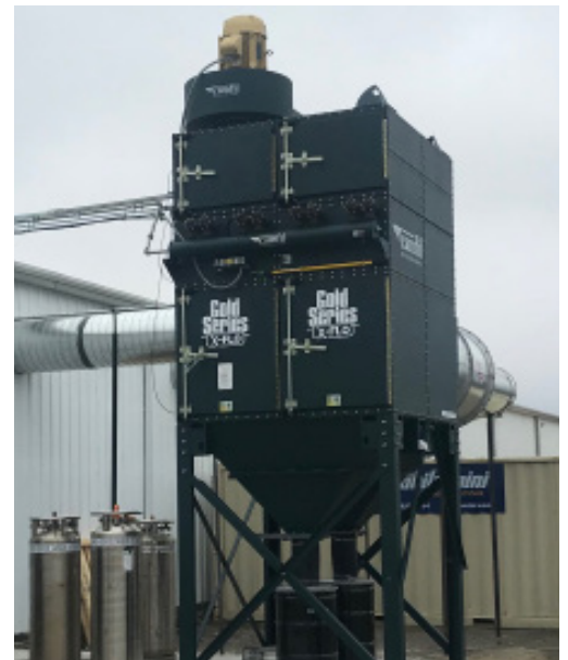
A GSX16 is frequently used to safely capture chemical dusts. An integrated safety monitoring filter is installed so that air can be safely recirculated back into the building without creating a combustible dust risk.
