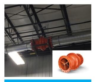
ISOLATION FLOAT VALVE Figure 3. The float valve can operate in the same or opposing direction as the conveying flow.
