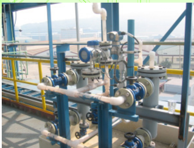
Figure 3. An Andritz facility opted to use electromagnetic flowmeters with virtual reference grounding in an extremely corrosive process that normally would require expensive corrosion-resistant rings.
