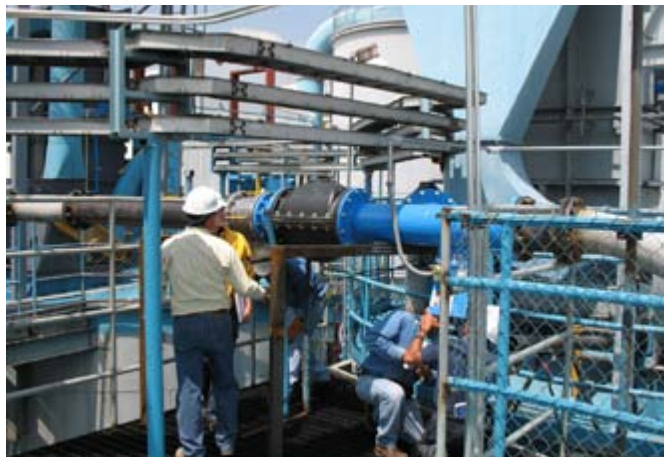
Figure 5. A 10-inch-wide pinch diverter valve directs material obstruction-free to two silos. The valve was configured to a specific angle of divergence to maximize flow, and came standard with double-wall construction for extended service life.
