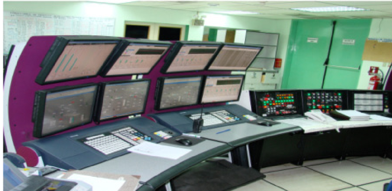
Figure 4. Experion PKS utilizes advanced HMIWeb technology, which provides an operator interface employing standard Internet technologies.
