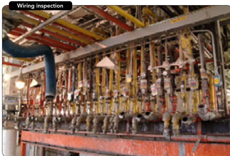
Figure 1. An initial inspection should verify safety barriers, wiring correctness and other conformance issues.
