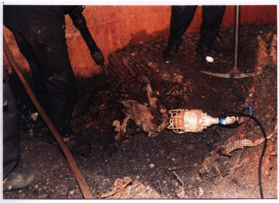
Asian Refinery Vacuum Tower Wash Bed
