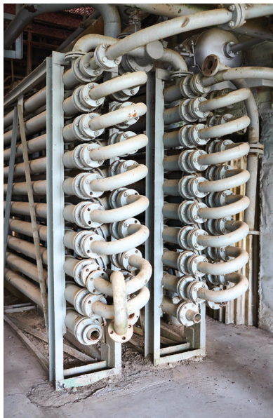
Figure 4. The hairpin heat exchanger includes end closures, which allow for thermal movements without expansion joints and the removal of tubes.
