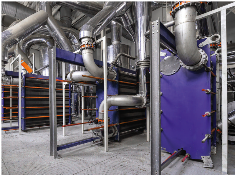
Figure 5. Plate-type heat exchangers help optimize thermal performance by enabling a number of close-temperature approaches and cross applications that previously were not economical or practical with shell-and-tube heat exchangers.
