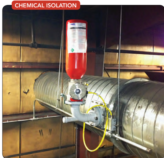
Figure 2. Extinguishant such as sodium bicarbonate smothers flame.
