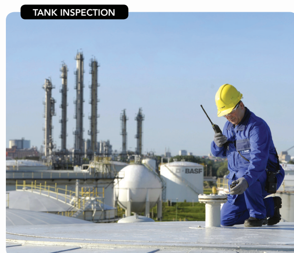
Figure 1. Plant technician uses a flame ionization detector to check seals and flanges on a set schedule. Source: BASF.
