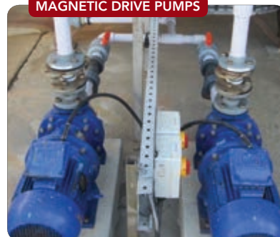
Figure 1. Such units are the most common sealless pumps used at chemical plants.
