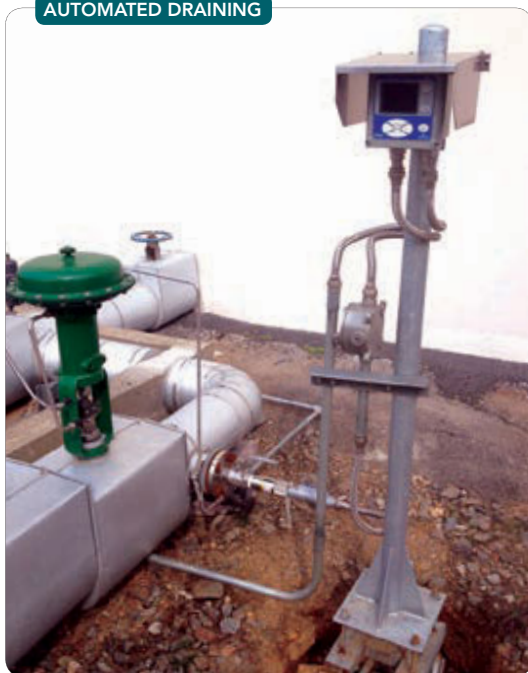
Figure 1. Loop-powered analyzer and conductivity sensor enable efficient removal of water from tank with minimal loss of naphtha.
