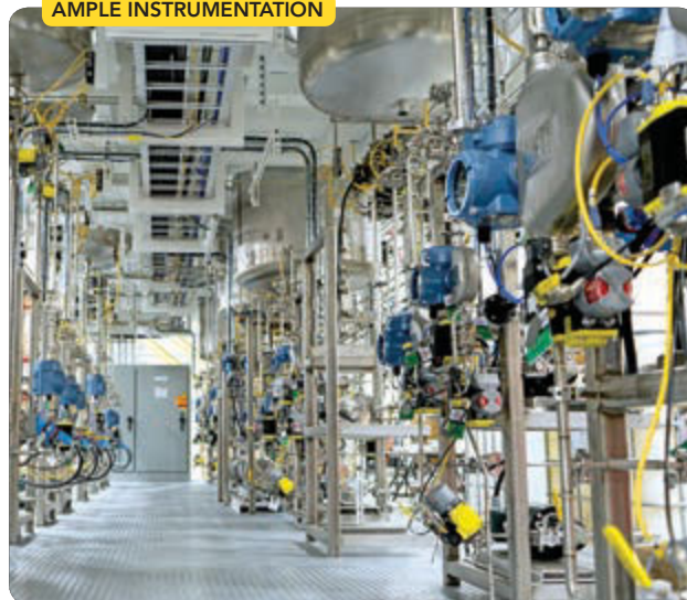
Figure 1. Because pilot plants usually are well instrumented, inadequate attention to calibration needs can markedly hamper startup. Photo courtesy of EPIC Process Systems.
