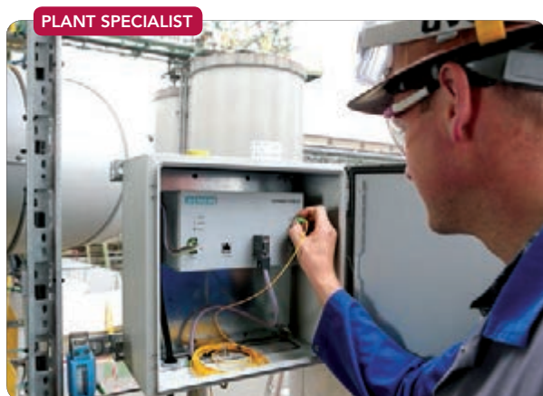
Figure 1. Matthias Hüning of Evonik plugs a glass-fiber coupler connected to the measuring probe into channel one of the transmitter.
