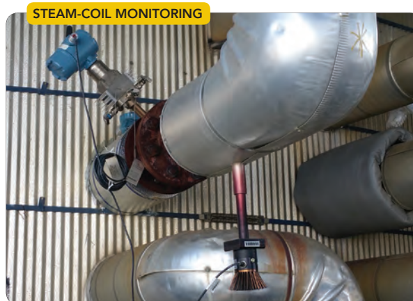
Figure 1. Teaming of wireless transmitter with energy harvester provided an ideal solution for gathering data.
