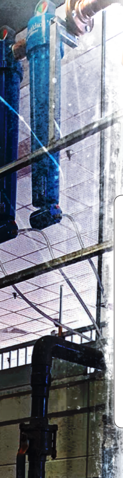
Figure 3. Such a unit drains automatically without loss of compressed air.
