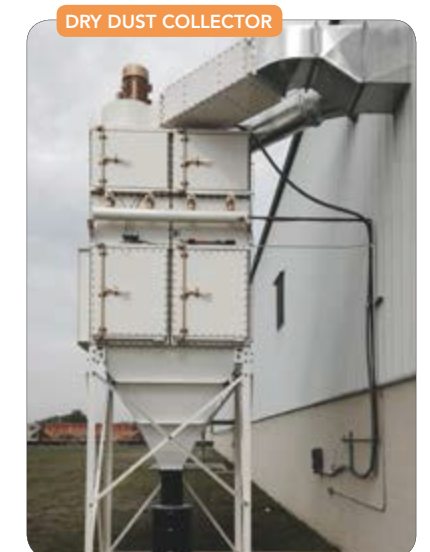
Figure 1. Positioning the collector in a location removed from the work area often makes sense.
