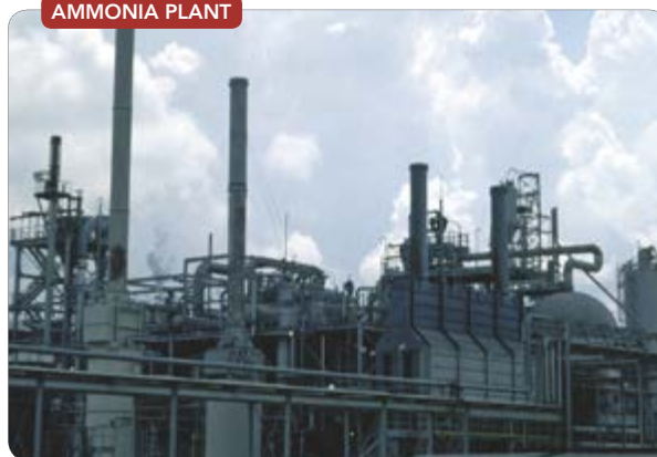
Figure 2. Issues with ion exchangers limited makeup water supply. Source: Suez.
