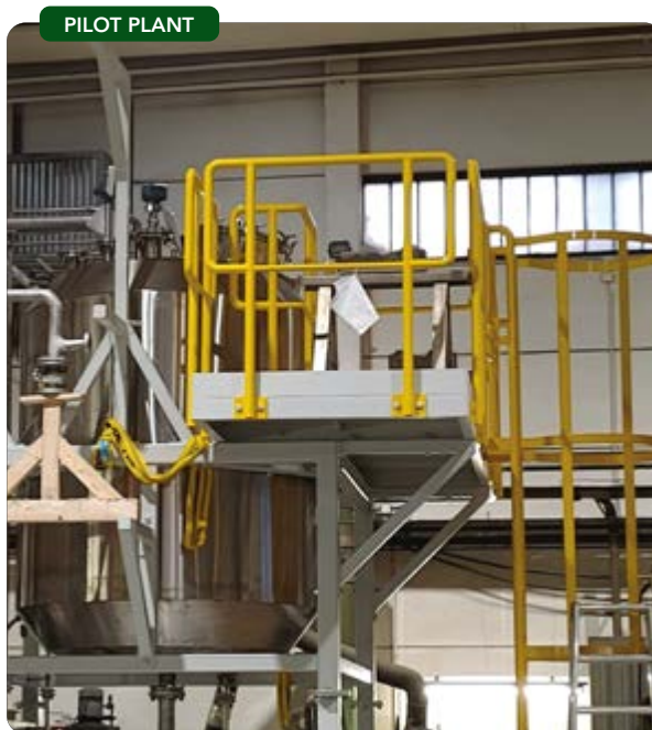
Figure 2. Work is progressing on 25-kg/hr unit in Germany. Source: MultiCycle.
