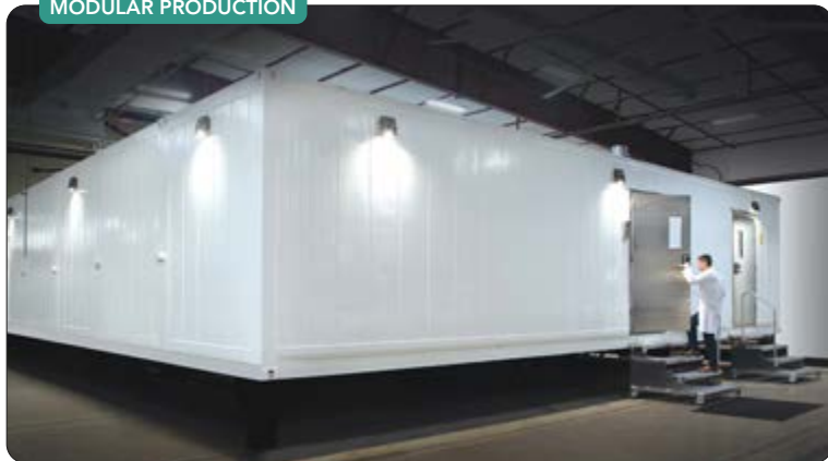
Figure 3. Off-the-shelf, prefabricated manufacturing facilities now are available for Biosafety Level 2 operations. Source: Cytiva.
