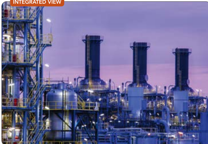
Figure 2. Looking at equipment reliability and overall process performance separately blunts benefits achievable. Source: AspenTech.
