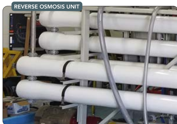
Figure 2. This technology can remove up to 99.5% of dissolved salts and impurities, and often serves as the final step in a treatment system.
