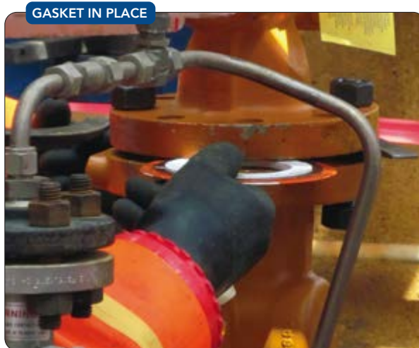
Figure 1. Proper flange separation allows for uninhibited insertion of gasket.
