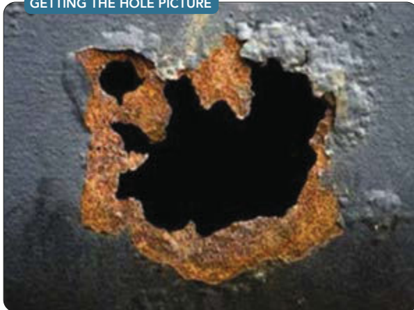
Figure 1. Alloy corrosion is one of many issues that modeling is tackling. Source: OLI Systems.
