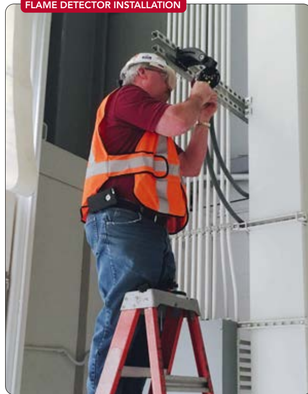
Figure 2. Proper placement requires avoiding obstructions between detectors and the area of interest.
