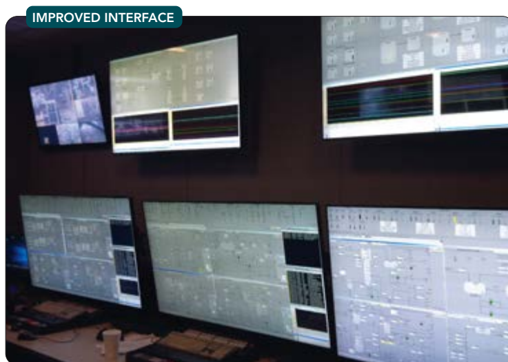
Figure 1. Control room displays now feature a high-performance human/machine interface that follows Abnormal Situation Management Consortium guidelines.
