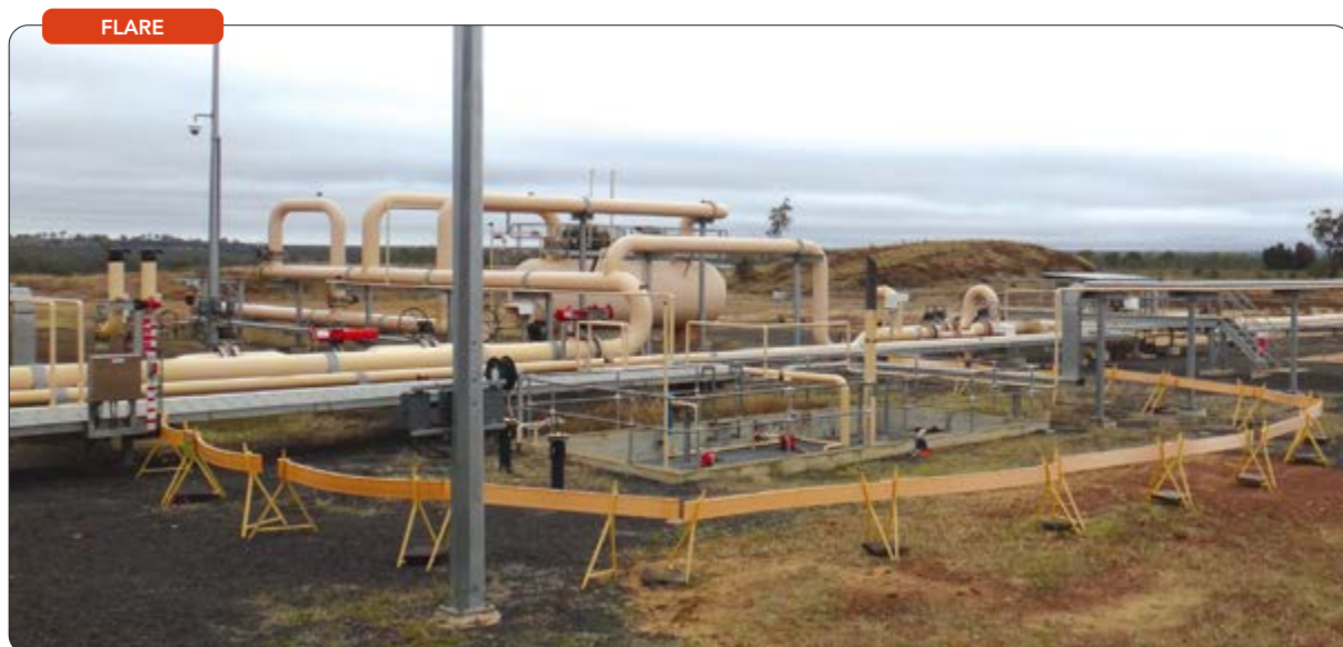
Figure 1. By burning released gases, unit provides an essential safety function.
