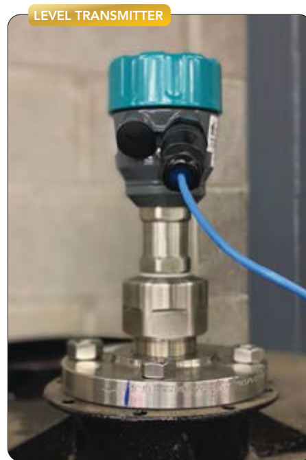
Figure 1. Guided-wave-radar device features power-over-Ethernet communications.
