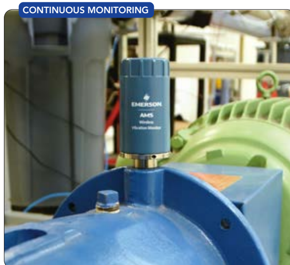
Figure 2. Small, easy-to-install sensors like this vibration monitor can warn if an asset needs attention well before a turnaround. Source: Emerson.
