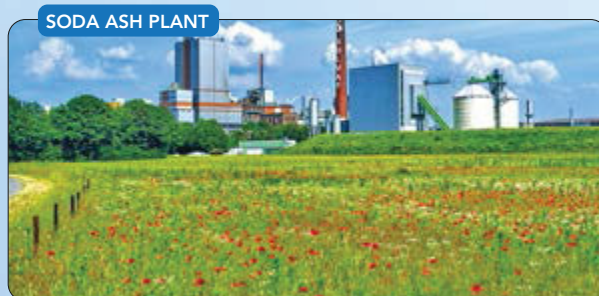
Figure 1. Project in Germany aims to make the unit the world’s first such plant powered primarily by renewable energy. Source: J. Kefferpuetz, Solvay Deutschland.
