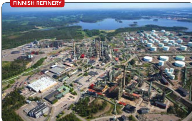
Figure 2. E. U. funding will support a green hydrogen and CO 2 CCS project at Porvoo site. Source: Neste.
