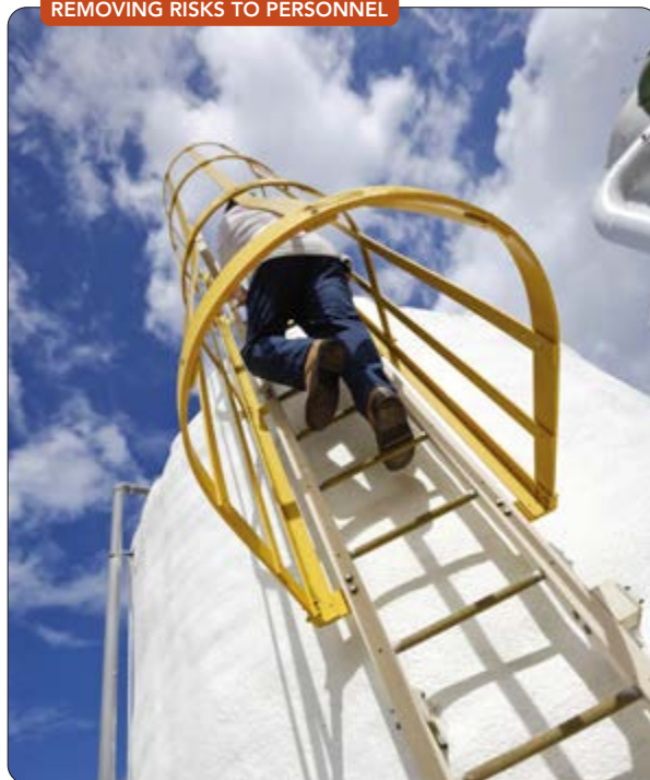
Figure 1. Remotely performing partial proof testing eliminates the need for staff to climb tanks.
