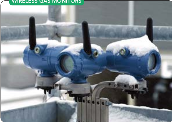
Figure 2. Available devices can withstand temperature extremes and exposure to the elements.
